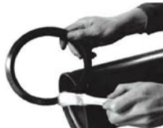
2.Lubricate gasket
