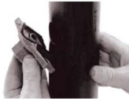
3.Gasket installation
